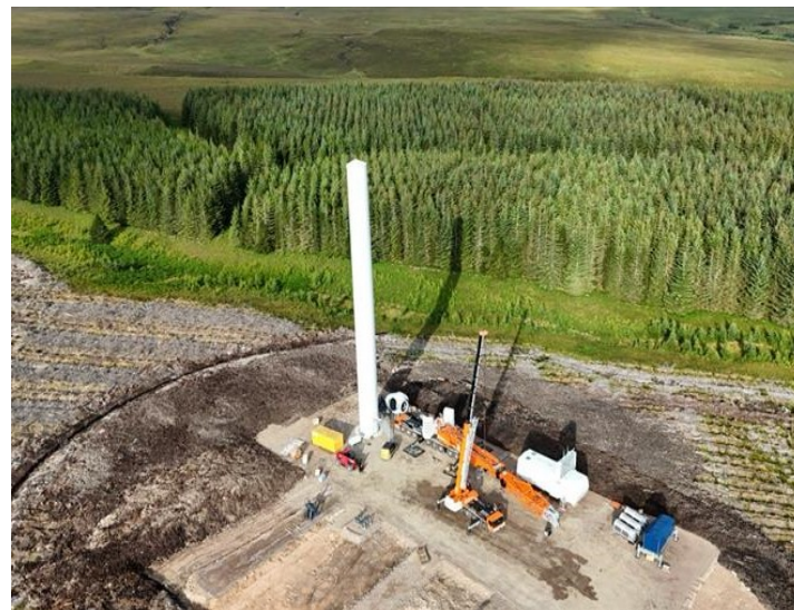
Installation of a turbine at the Limekiln wind farm in Scotland
