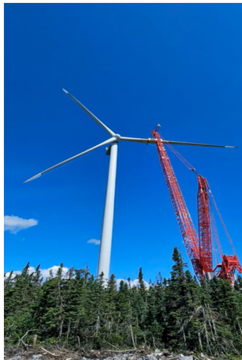
Installation of a turbine at Apuiat wind farm in Québec
