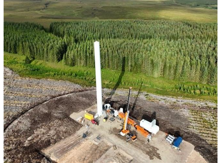
Installation of a turbine at the Limekiln wind farm in Scotland
