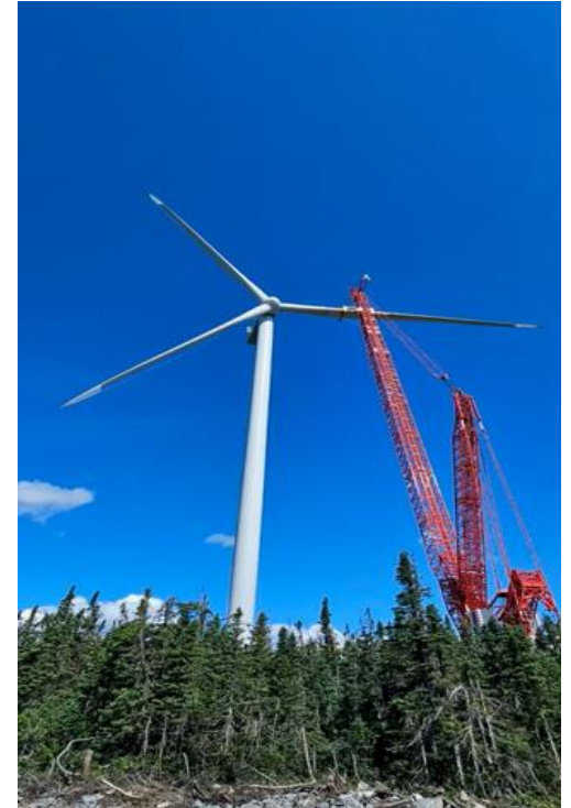
Installation of a turbine at Apuiat wind farm in Quebec
